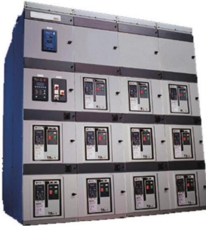
*Figure 3: An Arcflash Reduction Maintenance System shortens fault clearing times by bypassing time delays in the trip circuit.*
