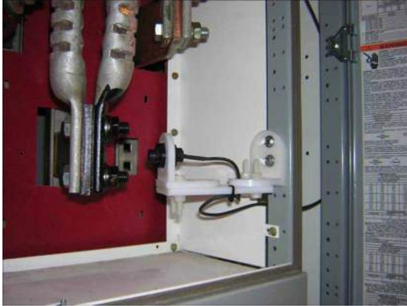
**Figure 4:** Pyrometers, like the one shown here, continuously monitor pressure junctions for signs of loosening.
