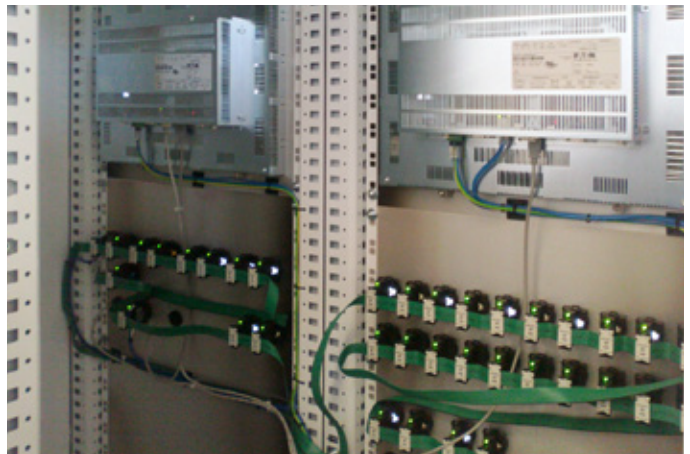
Lean Connectivity: XV400 touch displays with RMQ control circuit devices. The wiring effort can be reduced by up to 85%.
