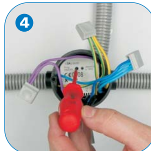
4 Activate the programming button a second time to finish the process (the LED and the connected lamp are switched OFF)
