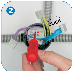
2 Activate the programming button (the red LED and the connected lamp are switched ON)
